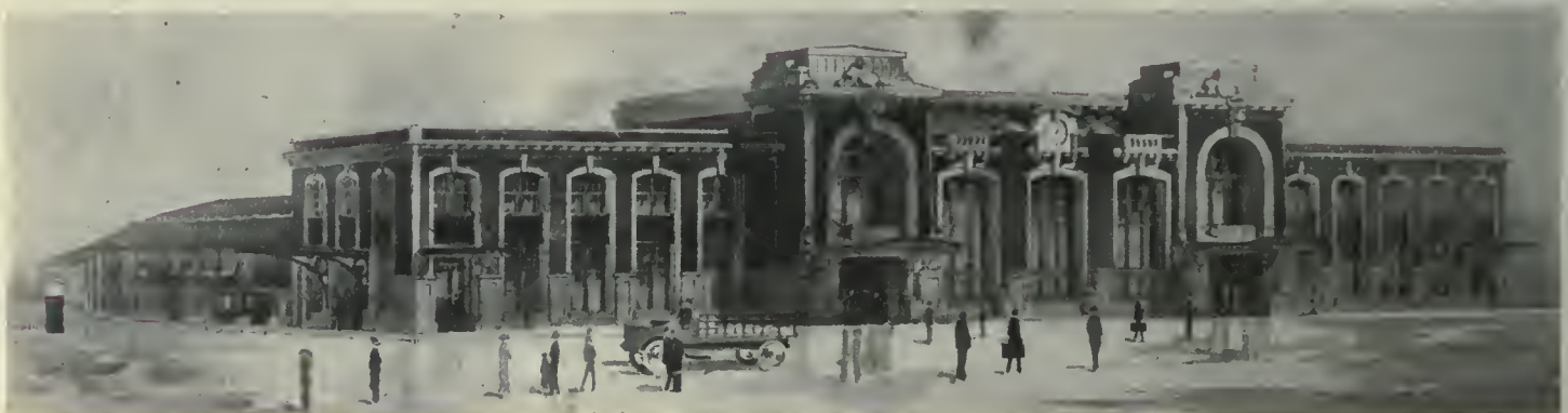
Handsome Building of The Great Northern Railway Under Construction on Reclaimed Area of False Creek Tide Flats, Vancouver, B. C.
